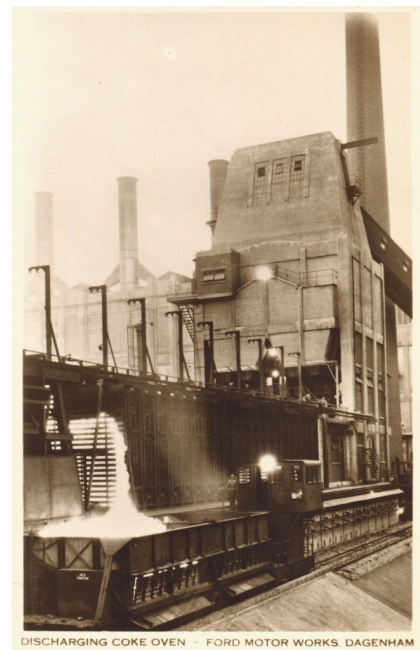
DISCHARGING COKE OVEN - FORD MOTOR WORKS, DAGENHAM
