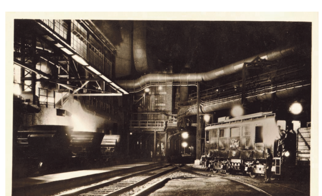
DISCHARGING SLAG IN LADLES - FORD MOTOR WORKS. DAGENHAM
